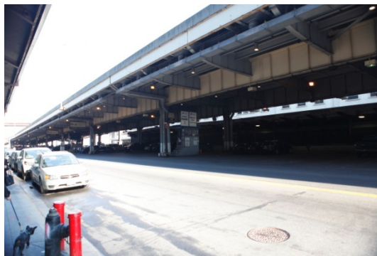
Figure 32 Existing Condition Under FDR Road
